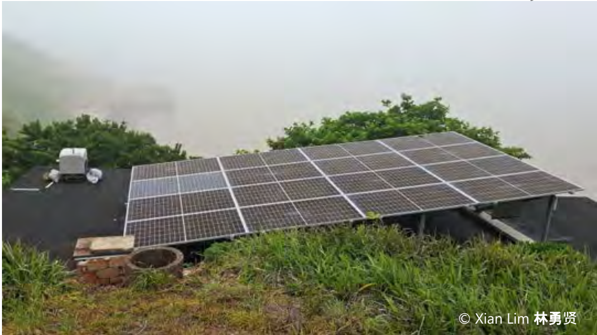
Plate 3: This photo was taken from the small grass-covered slope above the reservoir. The solar panels can be seen in the foreground, with the pier faintly visible in the upper left corner. May 2026.
