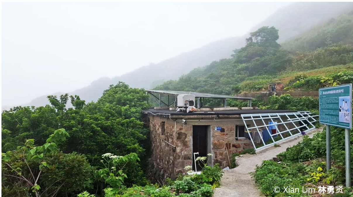
Plate 2: Volunteer Hut – the solar panels on the roof and the small grass-covered slope on the right are part of the water storage system. May 2026.
