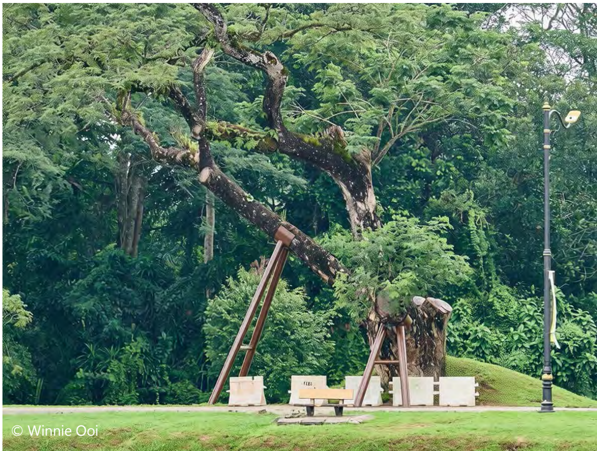
Plate 7: Rain Tree rehabilitated, Taiping, Perak, Malaysia, 21 Nov 2025.
